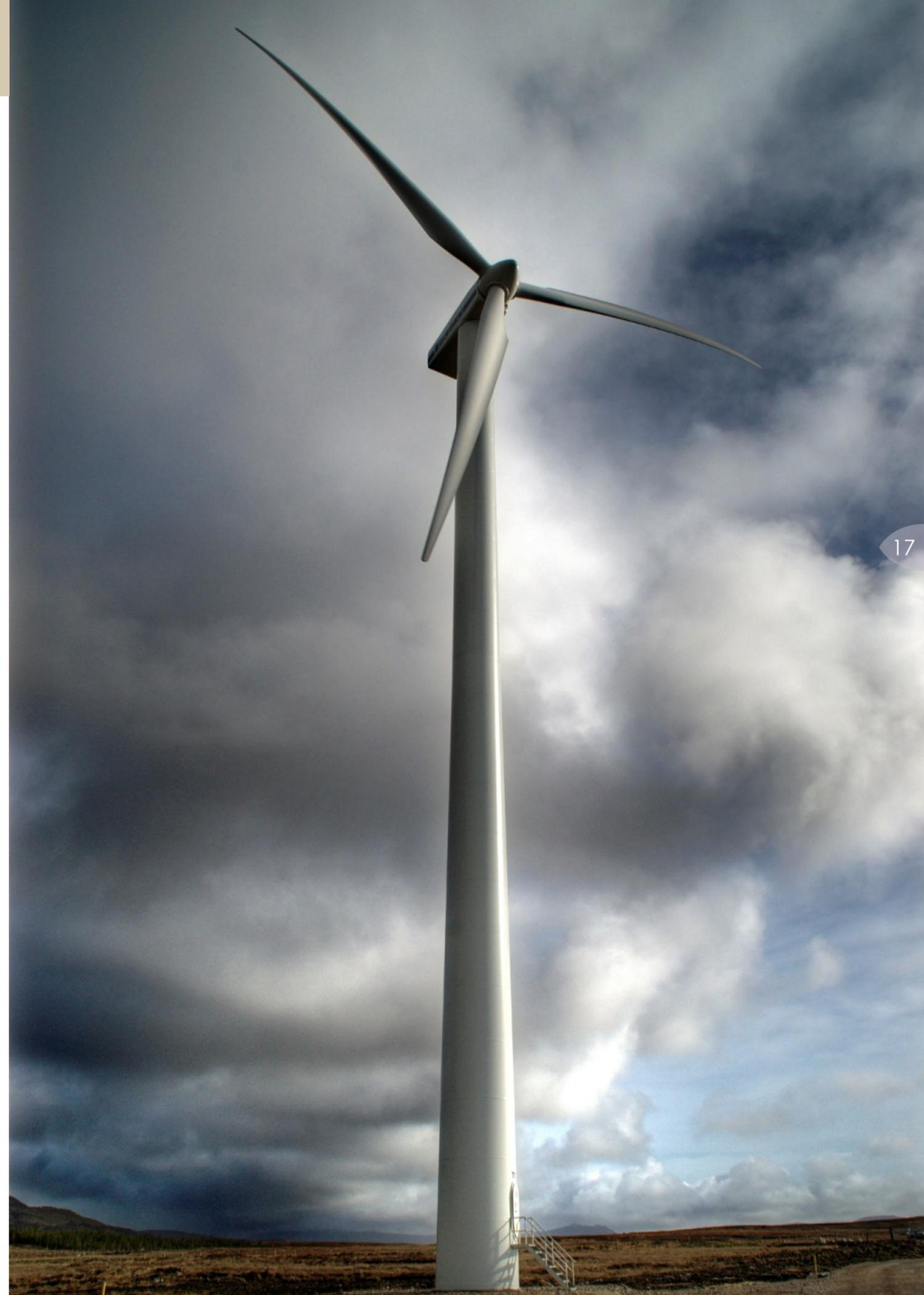
Noise is created by wind turbines as they rotate. The principle sources of noise are the turbine blades passing through the air and to a lesser extent the internal machinery such as the generator. Modern wind turbine blades are designed to minimise noise and the nacelle which houses the mechanical equipment at the top of the tower is sound insulated. Today's turbines are so quiet that it is possible to carry out a normal conversation while standing at the base of a tower.
