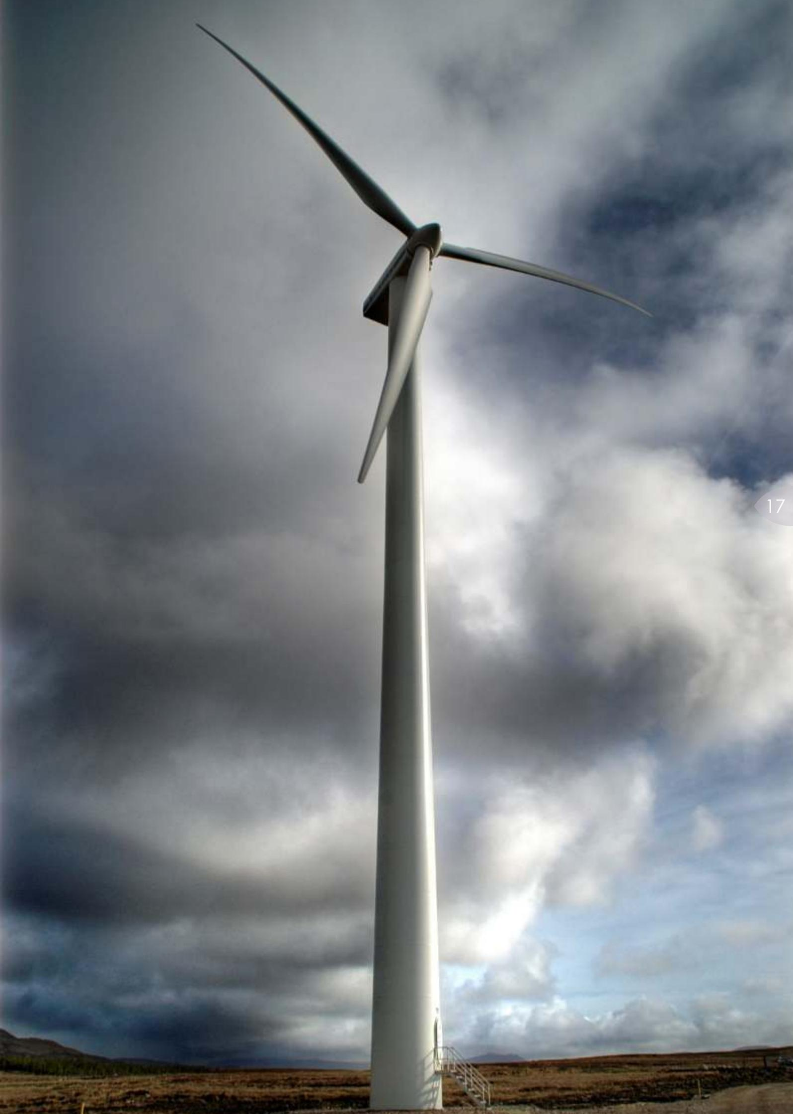
**W**ind turbines generate sound as they rotate - caused mainly by the turbine blades passing through the air and, to a lesser extent, the working of the generator inside the turbine. Modern wind turbines are designed to minimise sound emissions and the nacelle, which houses the mechanical equipment at the top of the turbine tower, is sound insulated. Today's turbines are so quiet it is possible to carry out a normal conversation while standing at the base of a turbine.
